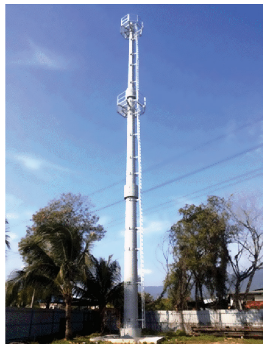
Figure 1. UHPFRC communication tower located in Malaysia
